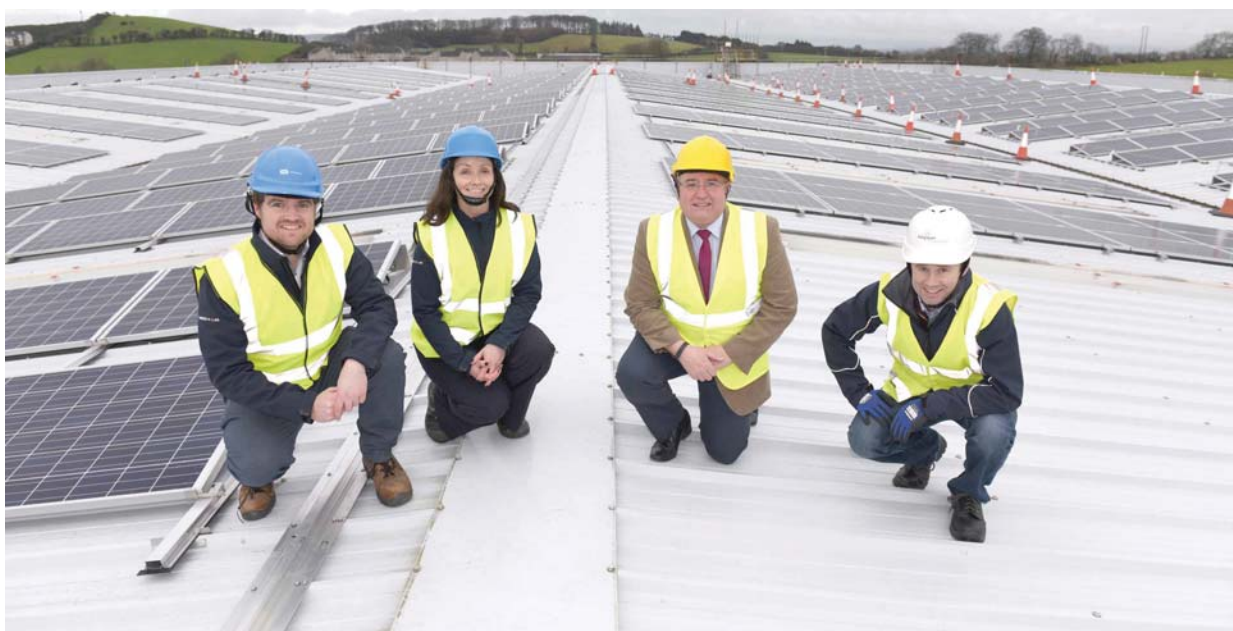
Rooftop Solar PV
