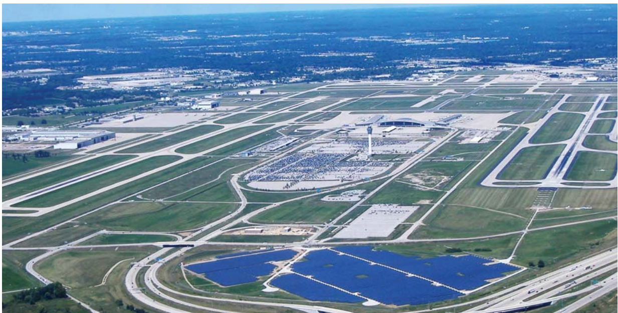
The IND Solar Farm at the Indianapolis International Airport. Image source: www.cenergypower.com
