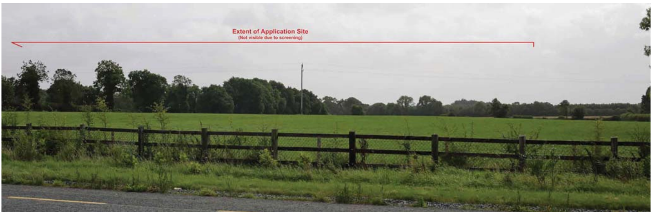
PL01: View from the North West along the R402 between Carbury and Johnstownbridge (2km from proposed development)
